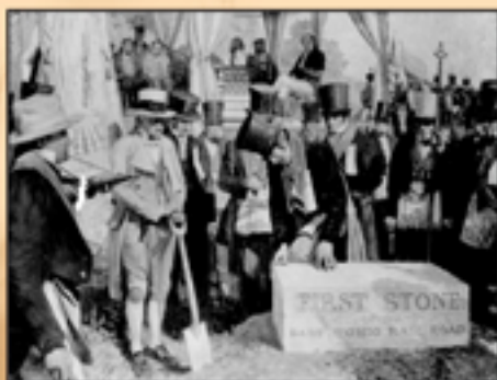
On July 4, 1828, Charles Carroll of Carrollton, the last surviving signer of the Declaration of Independence, dug the first spade of dirt to start construction of the B&O railroad.
